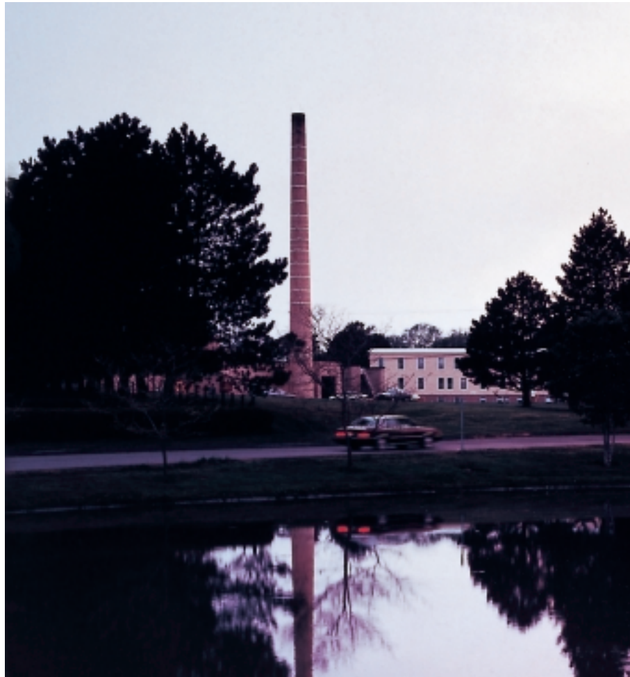
FIGURE 13 THE PRINCE EDWARD ISLAND HOME BOILER PLANT
