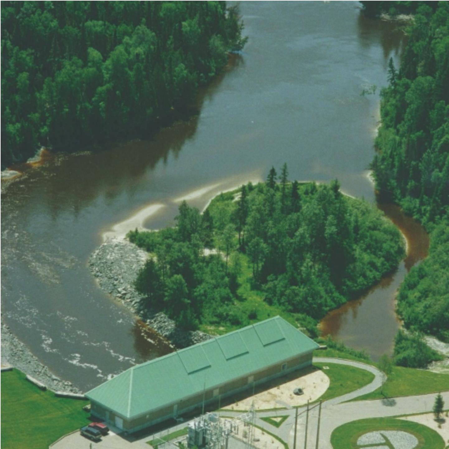
Wawatay Generating Station. Regional Power Inc.
